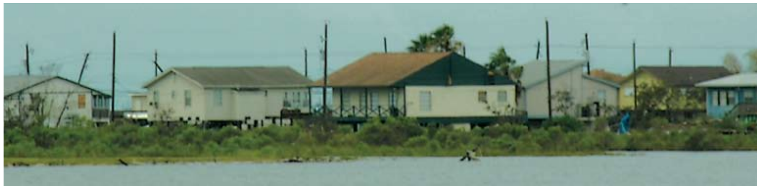
Figure 11: Galveston on the water – note lack of roof cover damage. The wind damage in Galveston was minimal.
