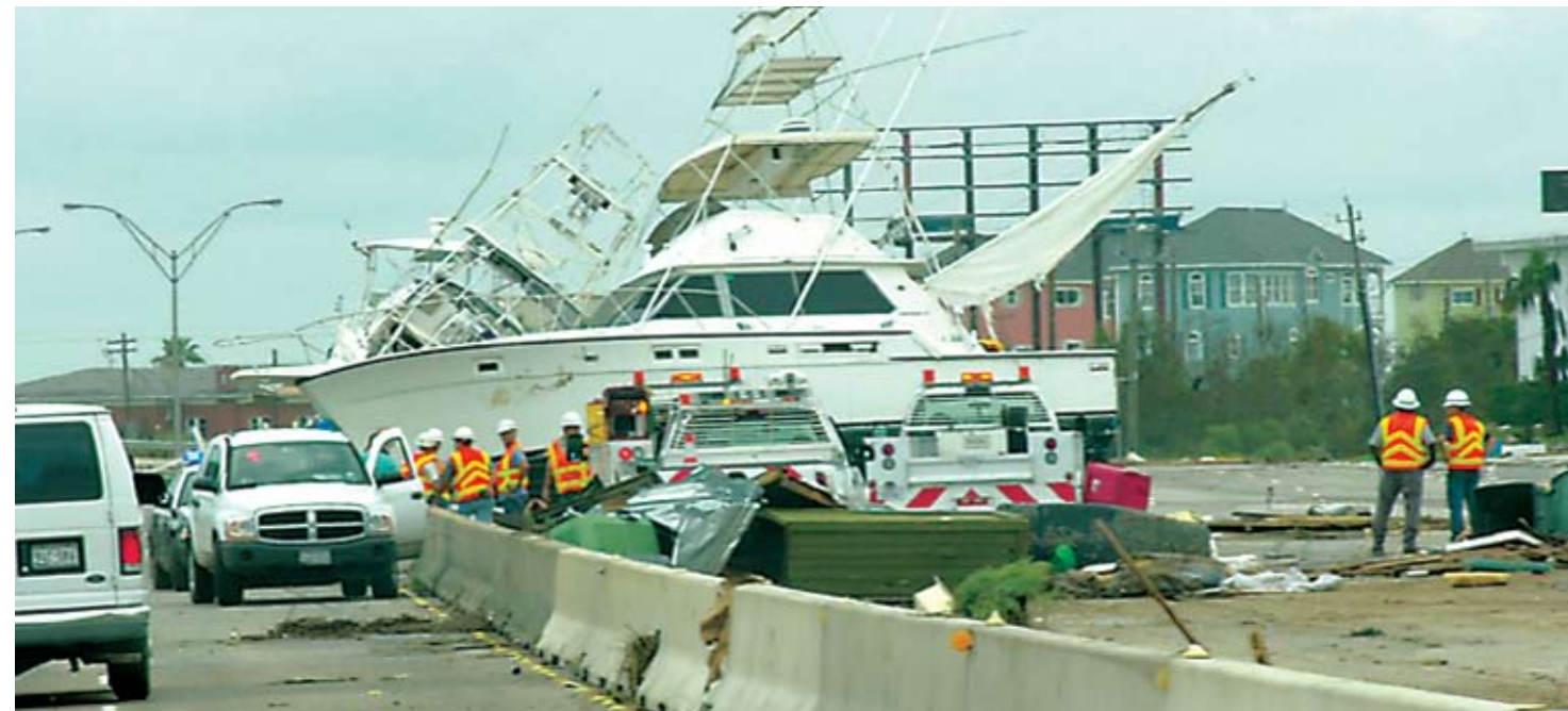
Figure 14: Damage and debris on highway leading to Galveston Island. Photo shows significant storm surge and still water flooding. Note the minimal damage on the roof covers of homes in the background. These roofs are 30 feet high, (i.e., two story house on 10-15 foot piles) and the minimal roof damage again attests to the low wind speeds of Ike.
