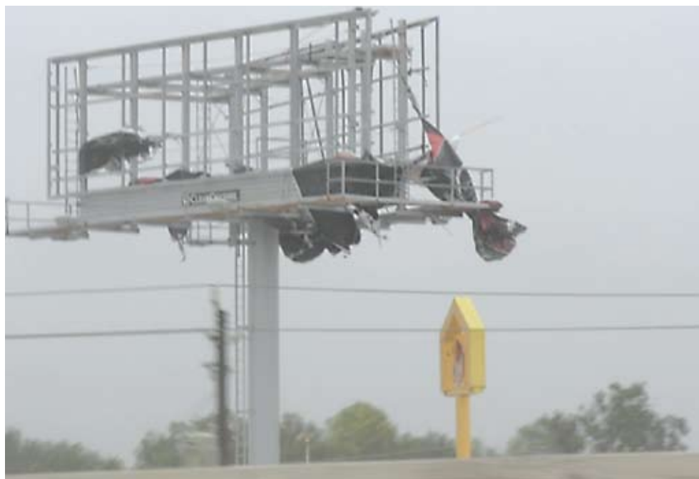
Figure 7: Commercial sign damage was heavy and was a significant source of debris in the Houston area.
