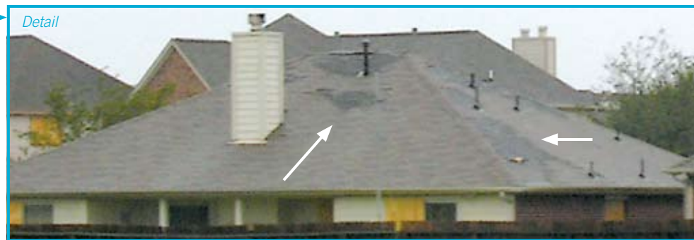
Figure 4 - A & B: Communities with mature tree canopies were observed to have less roof cover damage. Note the severe roof damage to the home visible on the far right of figure B.
